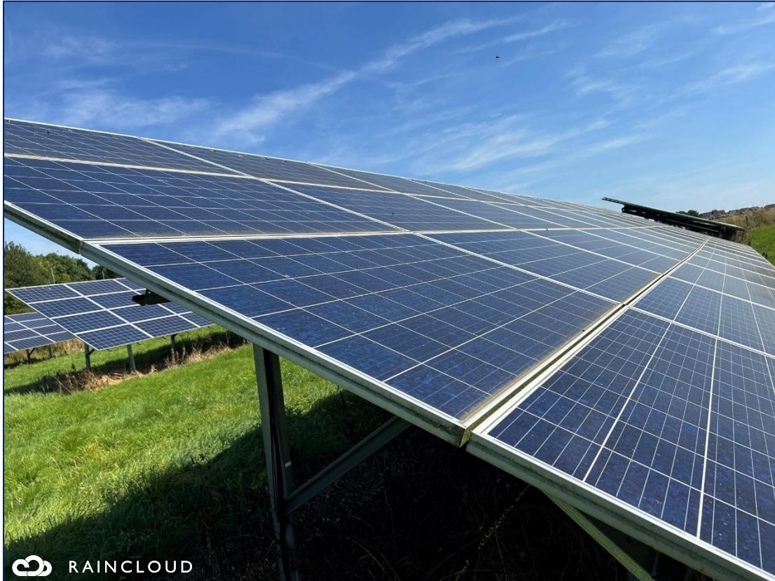
Plate A9.1. 37 18: Rainwater gaps on PV array table
